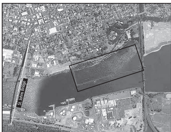
Left: Overhead shot of the area.
