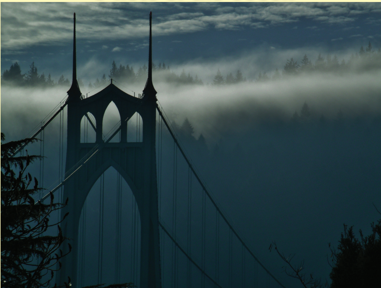
This gorgeous photo was taken by Paul Urban . Send your outstanding pictures of the St. Johns Bridge to be entered into the Review's photo contest.
