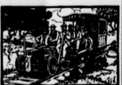
Edison Electric Locomotive Operated Experimentally at Menlo Park, 1880.
