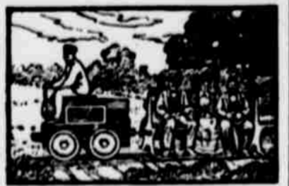
Edison Electric Locomotive Operated Experimentally at Menlo Park, 1880.
