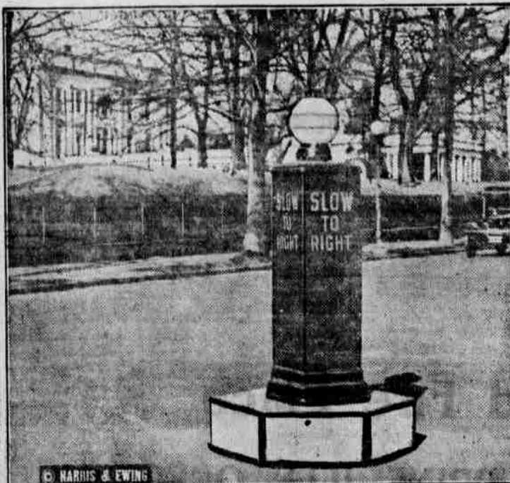
Flashing eighty times a minute day and night, this "silent policeman" equipped with an acetylene lamp directs the traffic in Washington near the southeast gate of the White House. The lamp throws a green light similar to those used along the Panama Canal. The White House can be seen in the background.
