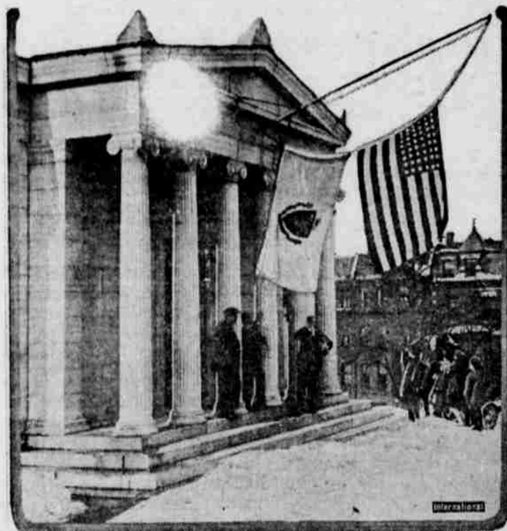
After an inspection of the Bunker Hill monument by the state engineers, the commonwealth of Massachusetts has formally taken over the care of the monument from the Bunker Hill association. It was found that the monument was badly in need of repairs. The photograph shows the Massachusetts state flag being hoisted over the entrance to the monument.
