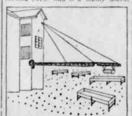
and labor saving arrangement. boom or arm to which the carrier is at tached must be strongly attached and guyed. The feeding racks are arranged in a semicircle that brings them just under the tip of the arm.
