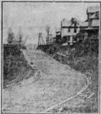
ROAD WITH DRAINAGE SYSTEM.
