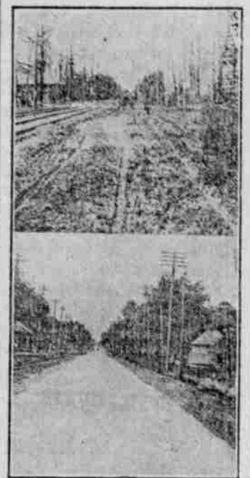
WAYNE COUNTY (MICH.) ROAD BEFORE AND AFTER USING CONCRETE.
