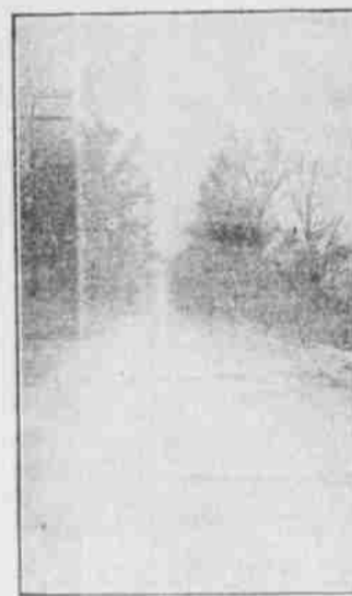
GRAVEL ROAD WELL MAINTAINED. [Courtesy Good Roads, New York.]
