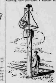
AUTOMATIC WARNING DEVICE. bolted to the regular tracks. To these are connected starting relays in such a manner that the trend of the wheels makes a contact as the car passes over, but there are no moving parts. The passing of a car over the contact making device simply starts the mechanism actuating the pendulum and gong, which, being provided with a timing element, runs a given length of time before stopping, thus warning all who approach .-- Popular Mechanics.
