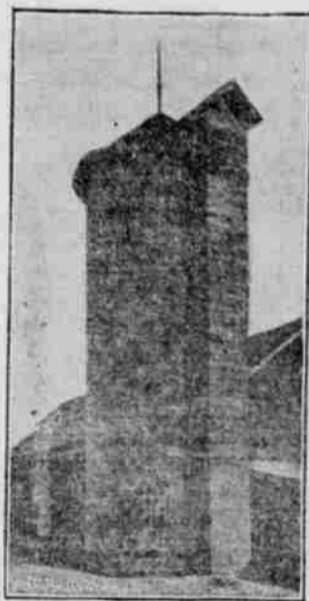
VITRIFIED CLAY BLOCK SILO.
