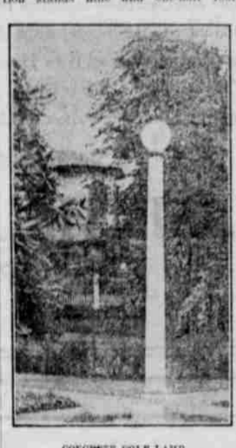
CONCRETE POLE LAMP. high, or just half as high as are the so-called 2,000-candle power arc lamps in the city streets. Each standard is a tapering shaft of granite white resting on a square base. There are no edgewise that can be broken off, and there is no part of the standards that can wear out. At the intersections of the streets the posts contain the names of the streets, the letters indicated, so that at nighttime there are no shadows cast by the lights. These street names can be as easily read at night as in the daytime. The burners are covered with frosted glass globes, which diffuse the light in such a way that all the walks and streets are adequately illuminated. The burners are sixty watt power, and it is estimated that if this plan of lighting were adopted for a more extensive use four or five of the burners could be used in place of one arc lamp with no increase in the amount of electricity used and with greatly increased efficiency. The standards adopted are such as a municipality could purchase for general use. Their cost is slightly in advance of the cost of an iron trolley pole, they are much more ornamental than the wooden poles to which are attached the arc lamps, and there is nothing about them that needs repairing except the tungsten lamps. The standards are admirably adapted for use in parks and parkways, and numerous towns have already placed similar standards in their parks. The placing of the light standards in a section laid out for residences, however, is a new one, and those who visited the place proclaim it a successful move.
