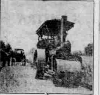
USING ROLLER ON COAL TAR ROAD.
