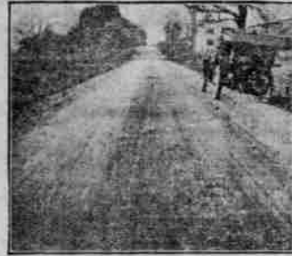
AN IDEAL HIGHWAY OF OIL AND GRAVEL [From Good Roads Magazine, New York.]
