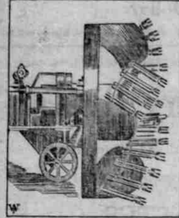
HEAD OF TUNNELING MACHINE.
