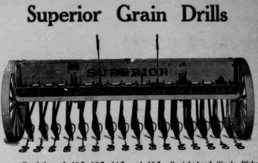
Consisting of 10-7, 12-7, 14-7 and 16-7. all right-hand Single Disks, with or without grass seed attachments. The effective feed method of lubricating the discs, style of discs and other good points all combine to make the SUPERIOR the best Seed Drill made.
