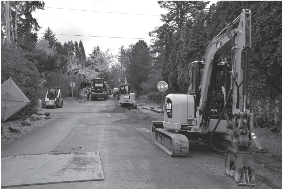
Keizer Public Works installs new water line on Joan Dr. in Keizer beginning April. Photo by CHARLES GLENN of Keizertimes
