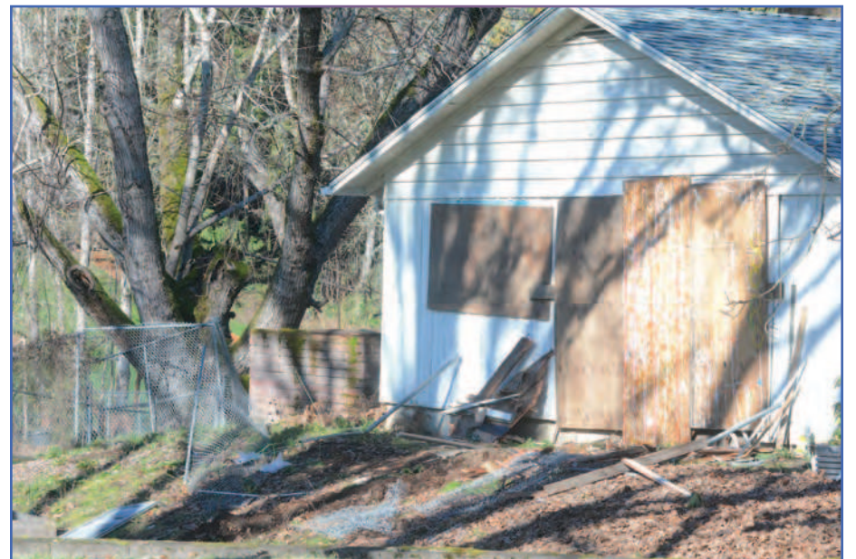
Where Modine's car went through the home is now boarded up, but the damage remains.
