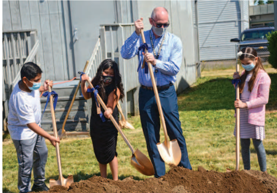
Kennedy students Jadiel Lopez (left), Abigail Ceja (second to left) and Madison Adair (right) join principal Jesse Leonard in breaking ground on construction at the school.
