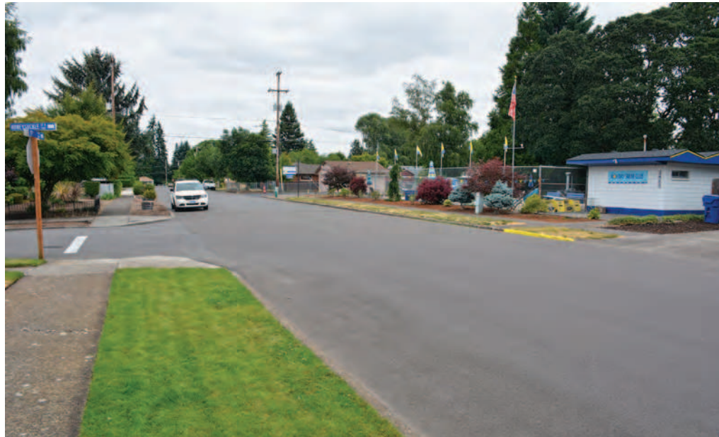
5th Avenue Northeast lacks crosswalks and adequate wheelchair access. The situation is turning hazardous as more people frequent the renovated park behind Holiday Swim Club.
