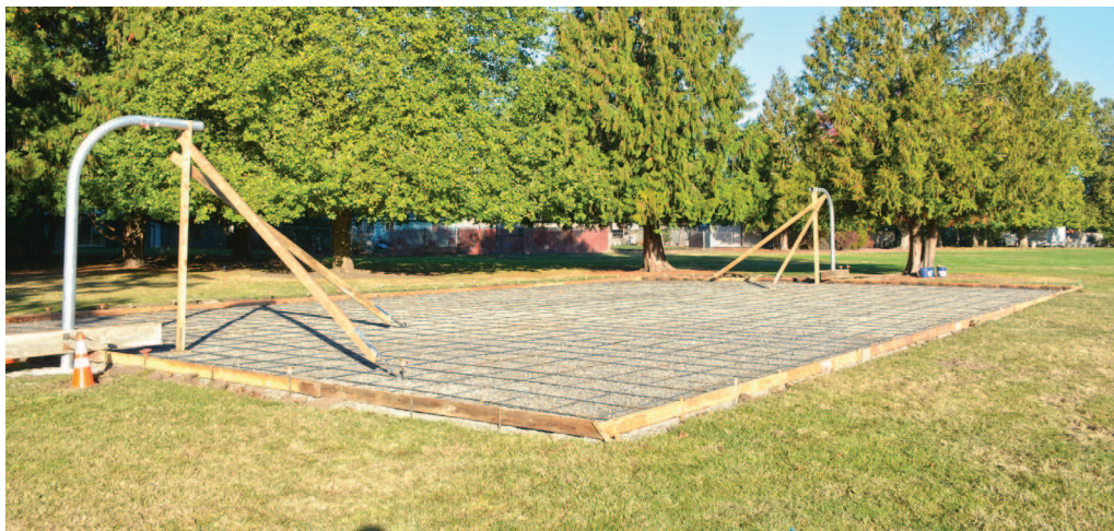
Keizer Parks Supervisor Robert Johnson said contractors were expected to pour a new full-size basketball court surface at Claggett Creek Park this week. KEIZERTIMES/Eric A. Howald
