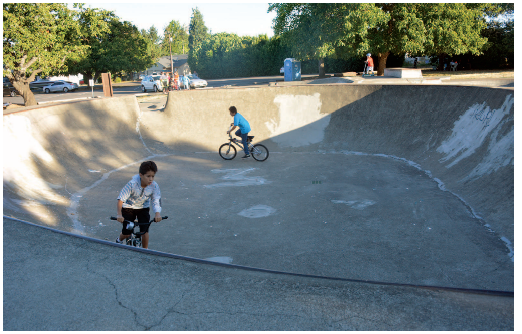
KEIZERTIMES/Eric A. Howald ABOVE: Cracks like the ones seen in the bowl of Carlson Skate Park are the reason the park needs to be resurfaced. RIGHT: Similar issues are affecting a basketball court at Claggett Creek Park.
