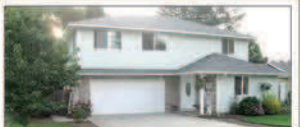
$239,500 4 BEDROOM - VALUE! 2002 built home with 2140 sf. Hardwood floors in main living area. Large kitchen & dining room area. Close to parks, schools & city center. (697495) Rick Maurmann 503.316.6330
