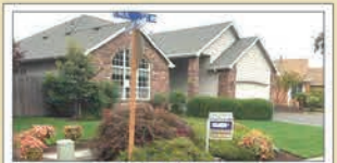
$319,000 BEAUTIFUL, WELL MAINTAINED Brick front, oak cabinets, vaulted ceilings, family rm & living rm, huge laundry rm. Walk-in closet in master, A/C, UGS. Private back yard w/shop building w/heat & elec. (695713) Charles Watts 503.884.0012
