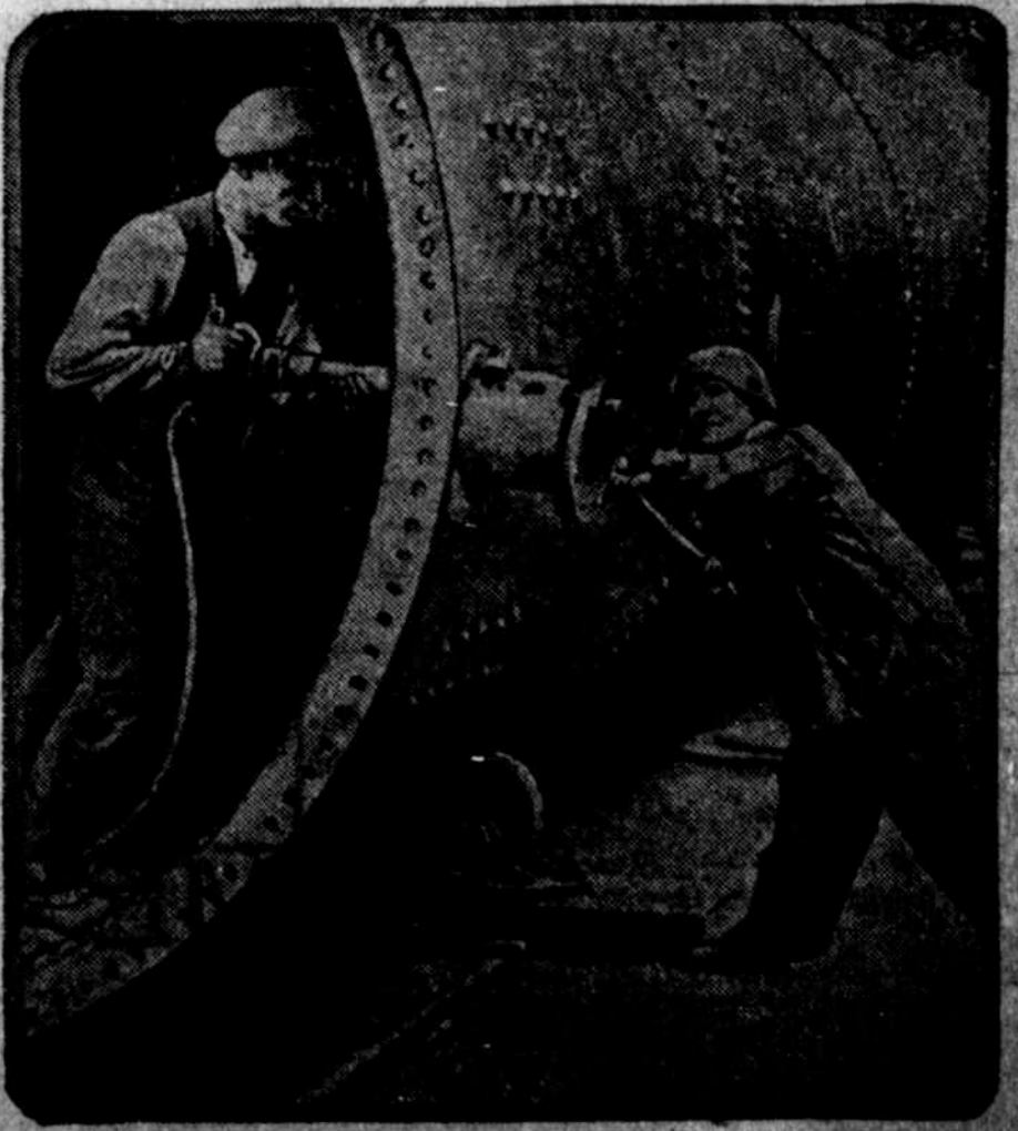
In a boiler factory in Glasgow many women have taken the place of the men who have gone to the front. One of them is here seen helping operate a hydraulic riveter.
