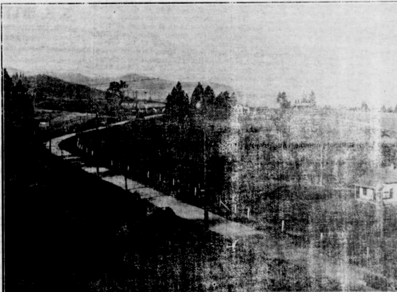
Asphaltic Concrete Road Constructed Between Talent and Ashland, Oregon, by Clark & Henery Construction Company.
