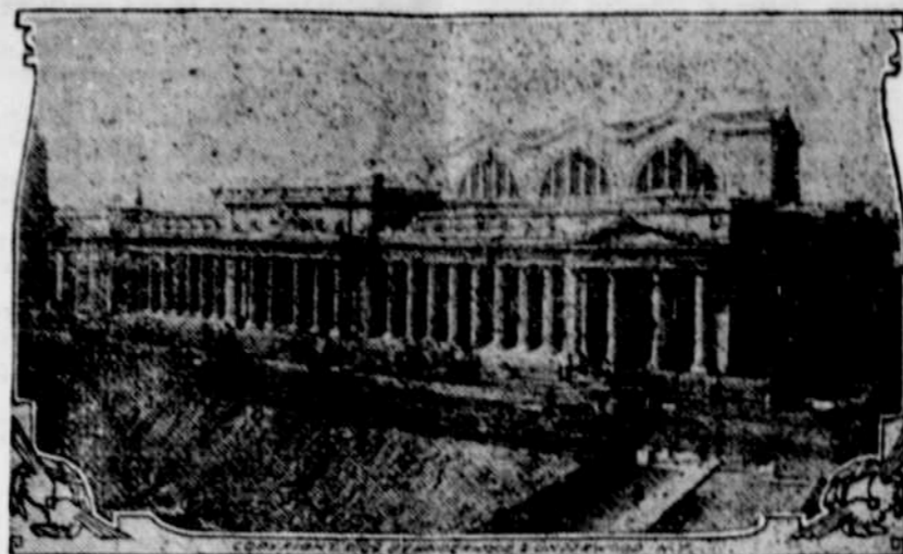
NEW PENNSYLVANIA STATION, NEW YORK, NEARING COMPLETION.
