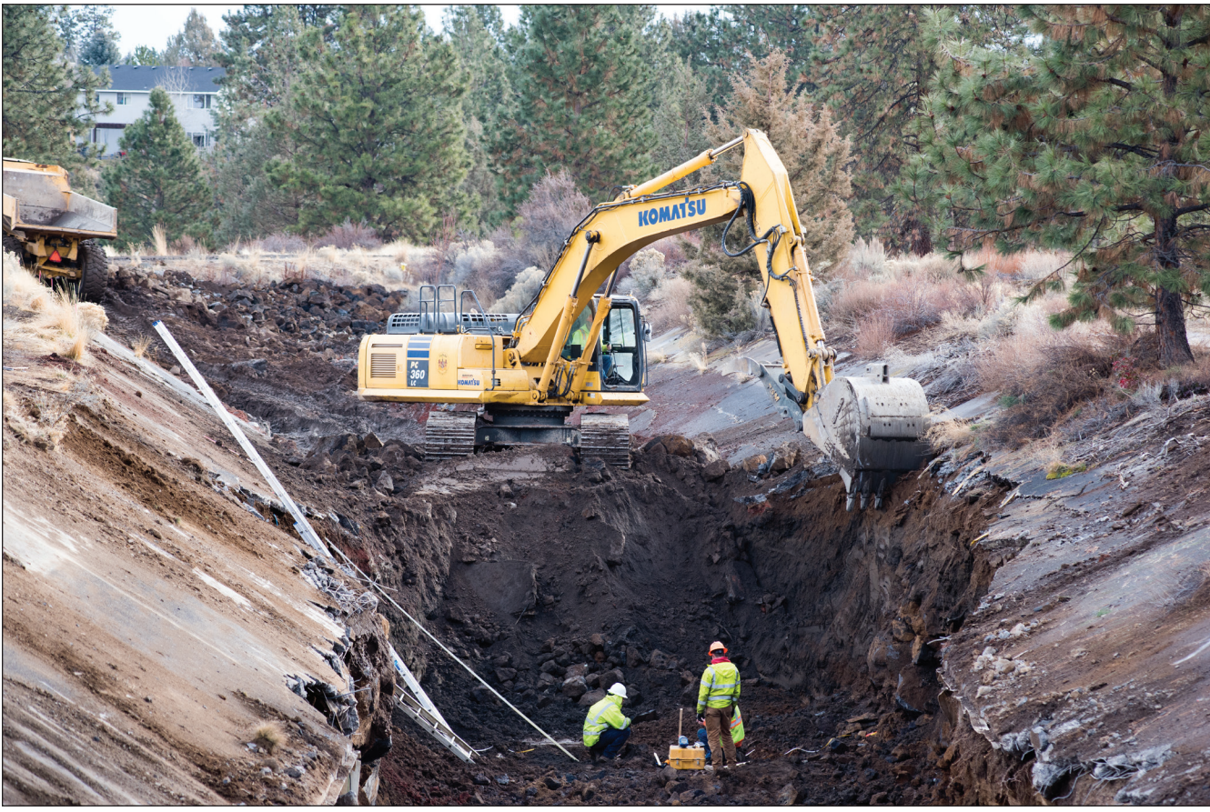
Photo provided by Central Oregon Irrigation District
