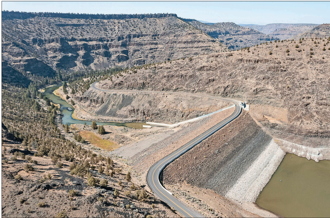
Water flows from Prineville Reservoir through Bowman Dam and into the Crooked River on Friday.
