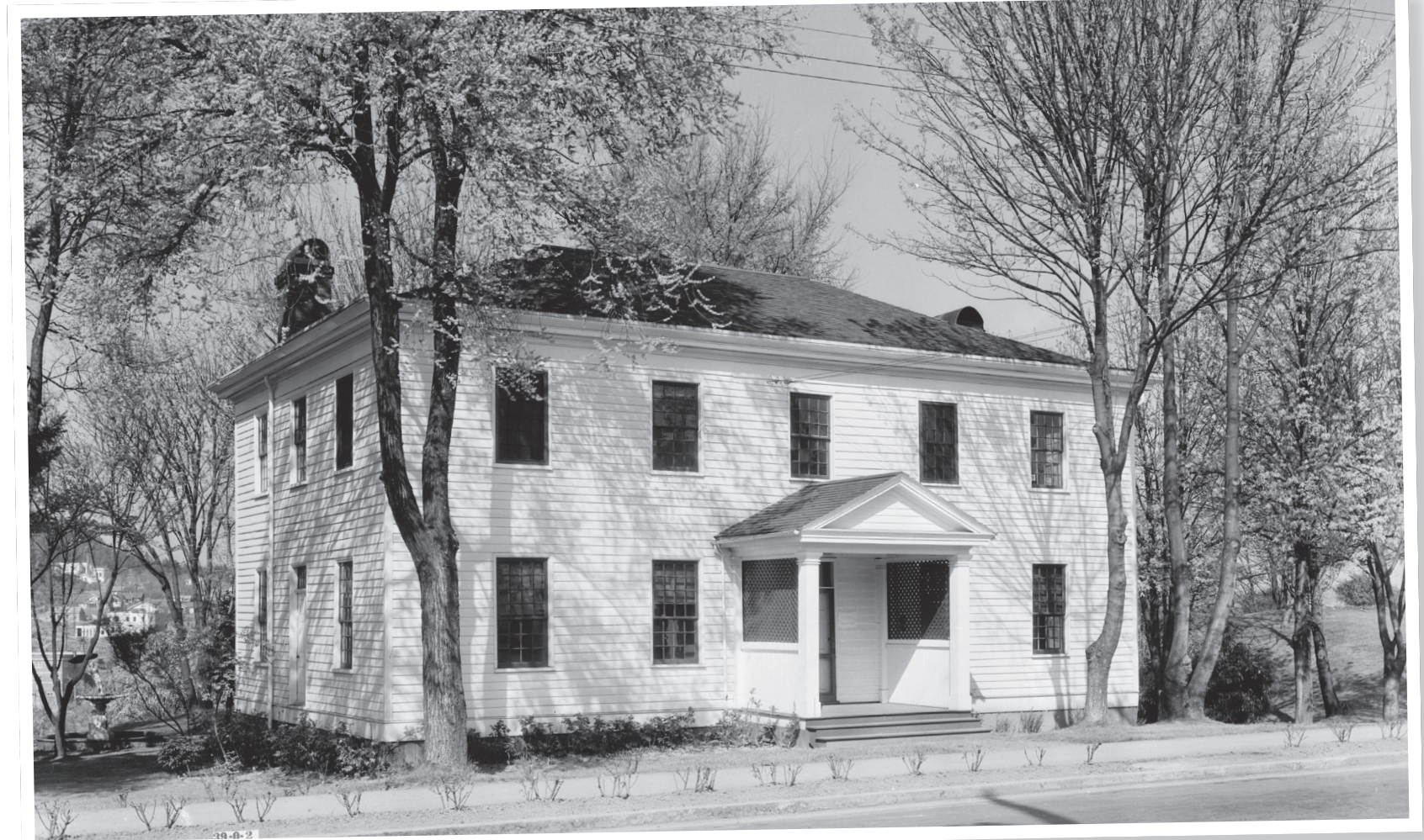
The John McLoughlin House was moved from Second and Third Streets in Oregon City.
