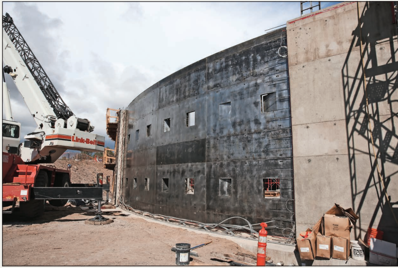
ABOVE: The interior of the 4 million-gallon reservoir at the South Redmond Water Facility, shown here May 26, will be fed by a 983 foot deep well. LEFT/BELOW: Several layers of material are used to construct the walls of the reservoir.
