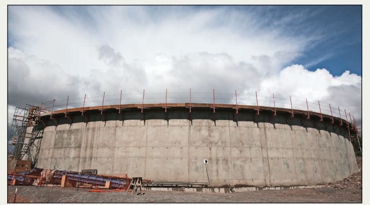
ABOVE: The interior of the 4 million-gallon reservoir at the South Redmond Water Facility, shown here May 26, will be fed by a 983 foot deep well. LEFT/BELOW: Several layers of material are used to construct the walls of the reservoir.
