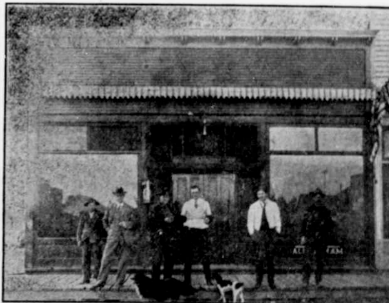
Exterior view of A. G. Allingham's Buffet, Redmond
