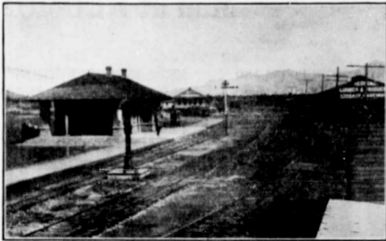
Stone Union Depot at Redmond used by Oregon Trunk Ry. and Oregon-Washington Railroad & Navigation Company
