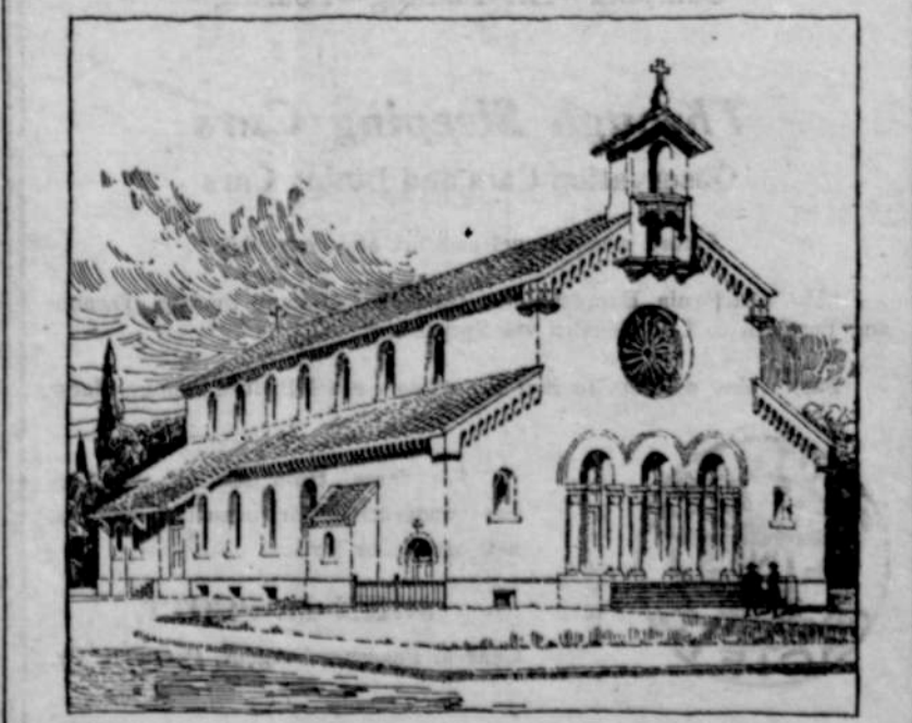
NEW ST. PETER'S CHURCH, PORTLAND, FOR WHICH EXCAVATION HAS BEEN COMPLETED
