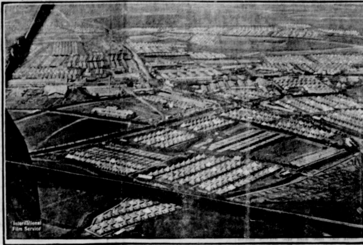
A remarkable photograph of Camp Pontanezen at Brest, France, through which all American soldiers embarking for home at that port pass, made from a French dirigible. The camp is the largest of its kind in the world. There are 60 miles of duckboards in it, and housing accommodations for 80,000 men at one time.
