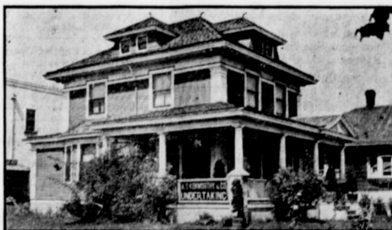
BRANCH OFFICE, 4615 66th St. S. E., at Arleta Station
