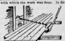
ing it the chain was anchored to a window sill or studding. The handle of the cant hook was placed against a flooring board and the hook caught into a link of the chain. The handle was then pulled back, forcing the looring boards into place. When doing this a block should be placed between the hook on the chain and the window sill and also between the cant hook ent of Missouri Valley Farmer.
