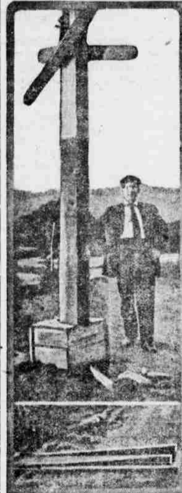
Highway Block Signal and the Trap at the End of the Dangerous Stretch Which Operates It.
