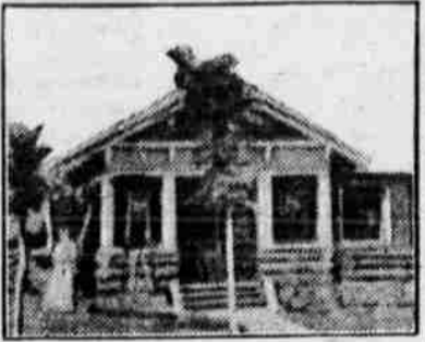
In This Pretty Bungalow the "Logs" Are Precast Concrete Units, Laid Up With Mortar, Like Any Masonry, and Stained Wood-Brown on the Outside to Look Natural.
