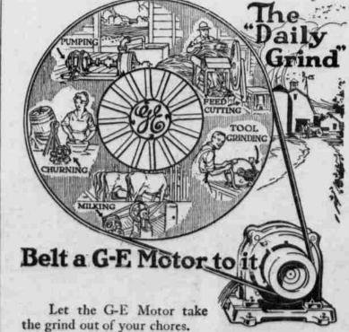
Motor-driven machines will milk, separate cream, churn, grind tools, pump water, cut feed and ensilage, grind and shell corn, split and saw kindling, thresh grain and perform practically all ordinary tasks requiring steady application of power. A G-E motor will soon pay for itself in labor and time saved.
