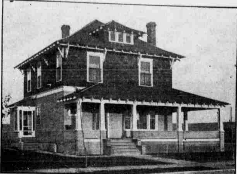
Residence of E. R. Hamilton just Completed at cost of $3,500
