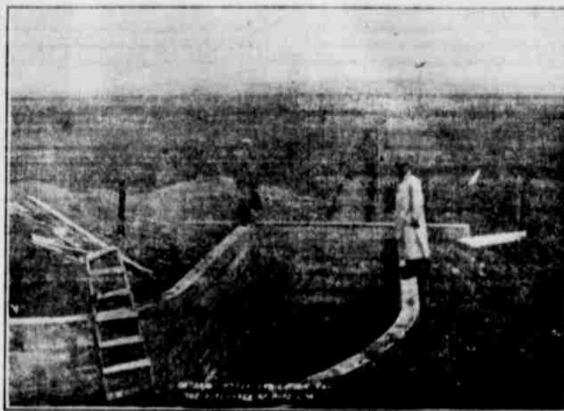
HEADGATE OF ONTARIO-NYSSA IRRIGATION PROJECT
