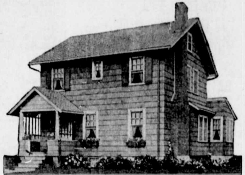
This attractive colonial home is distinctive without being extreme; it bears the test of good taste, right principles. The floor plans are conveniently arranged, each room being allotted ideal dimensions.
