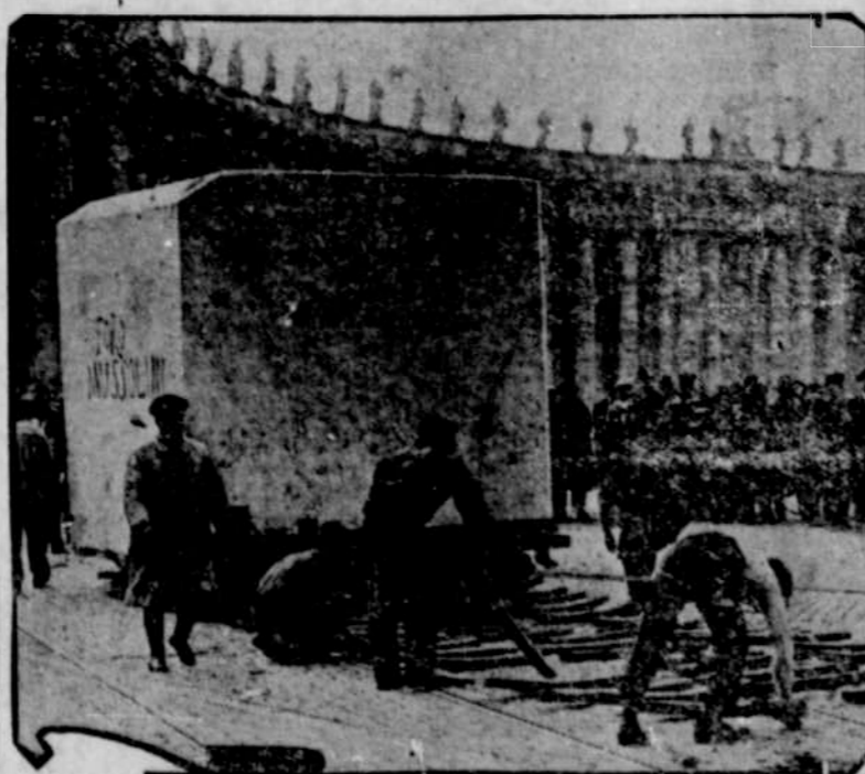
Here are eighty-six tons of marble being moved through St. Peter's square in Rome. It is the giant block which will serve as a base for the lofty monolith in the new Mussolini stadium which is under construction. Curved strips of soaped wood were used to transport the heavy block.
