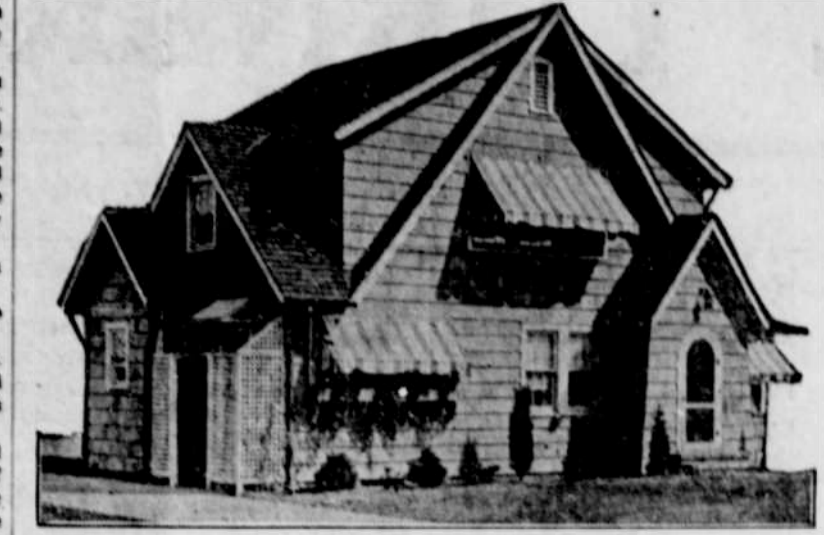
The roof lines and window arrangement in this house with the numerous gables give it a very unusual and attractive exterior appearance. The dimensions are 24 feet by 29 feet. There are six rooms and a good-sized sun porch. One bedroom on the ground floor is a convenience.
