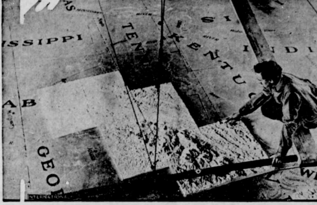
Le Roy Nichols, map engineer, placing one section of the largest relief map in the world, being constructed in a special map house in Babson Park, near Boston. The map, constructed of special gypsum blocks, will be 65 feet long and 46 feet wide and will follow the curvature of the earth.
