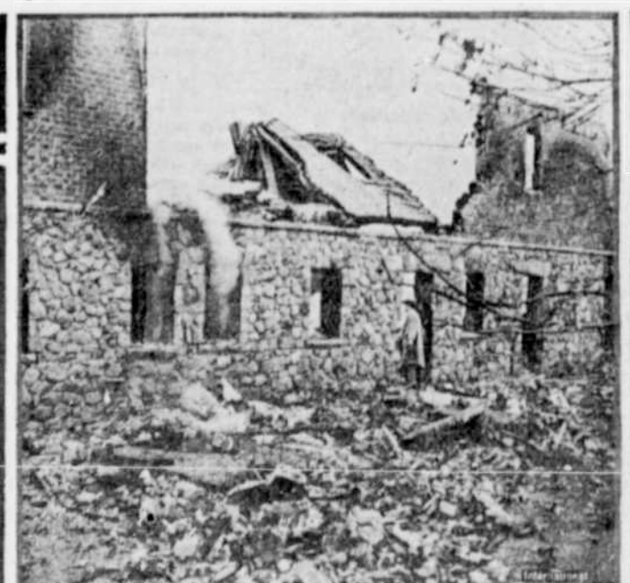
Ruins of orphanage at Peapack, N. J., conducted by Baptistine Sisters of the Nazarene, which was burned recently. Of the 79 children in the building, only three were killed, the others being carried out by two sisters at the imminent risk of their lives.
