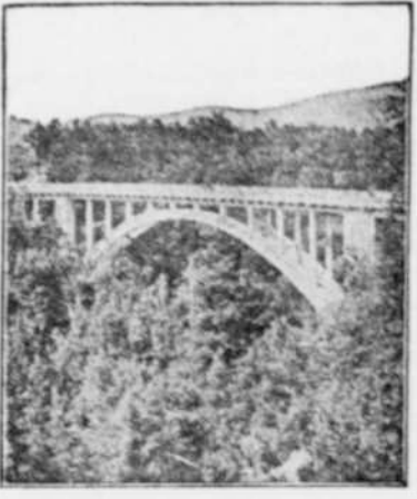
A Modern Concrete Structure.
