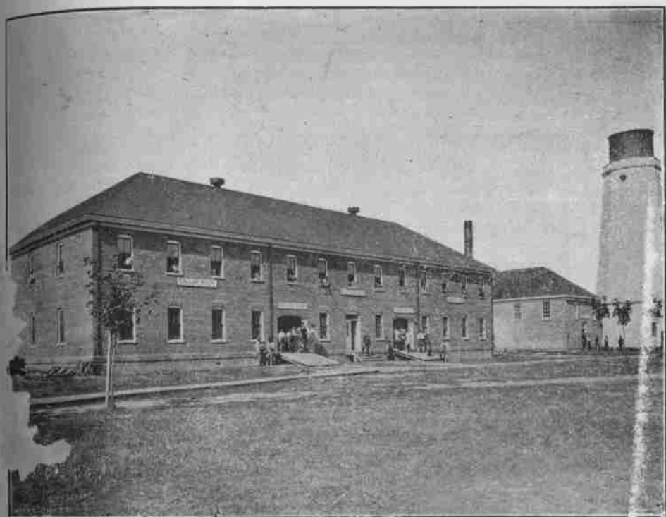
INDUSTRIAL TRADES BUILDING AND WATER TOWER.
