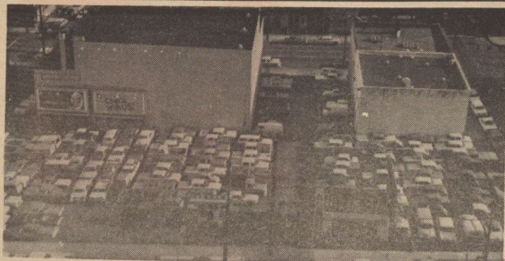
THIS CITY BLOCK IN DOWNTOWN PORTLAND is the site of a proposed parking facility for employees at the State Office Building. The three buildings will be razed and a five story structure will be constructed with parking spaces for 500 cars. The block is bounded by Columbia, Clay, Third and Fourth Streets.
