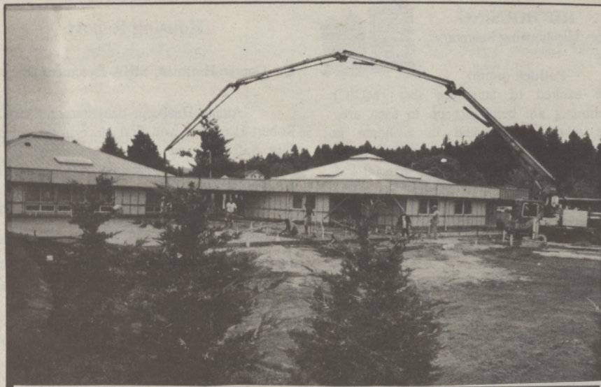
Pouring concrete for the foundation of the new addition.
